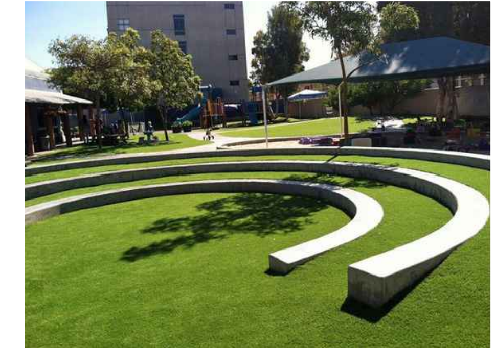
Seatwall - Cast In Place Concrete
