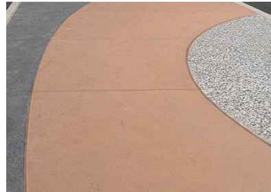
Coloured Concrete Paving
