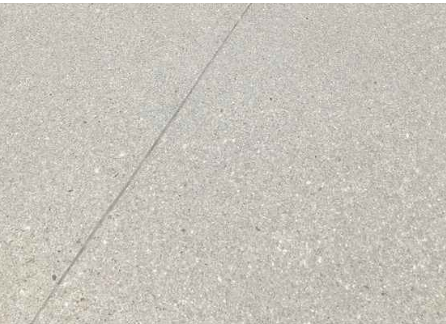
Standard Concrete Paving
