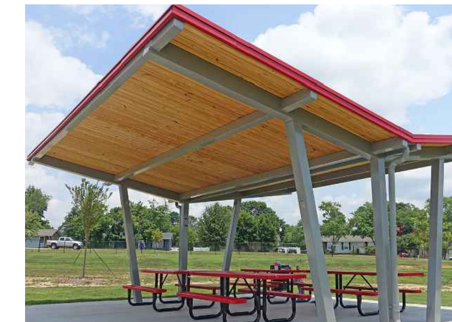
Gullwing Shade Structure
